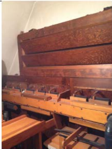
Figure 1: The two horizontal swell shutters. The vertical are below and cannot be seen here. Note that these shutters are WIDE OPEN and do not allow much sound out into the church. The large horizontal box below them is the swell motor mechanism.
