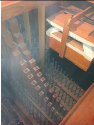
Figure 3: At the right is the air reservoir for the swell motors. Below are the smaller pipes. The square pipes are the 8' Flute.
