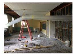
By Thursday, the bathroom wall was knocked out, and this filtration unit was set up. Asbestos in the carpet and ceiling glue was slated for removal today!
